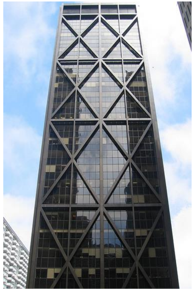
A Cross Braced Building in San Francisco
